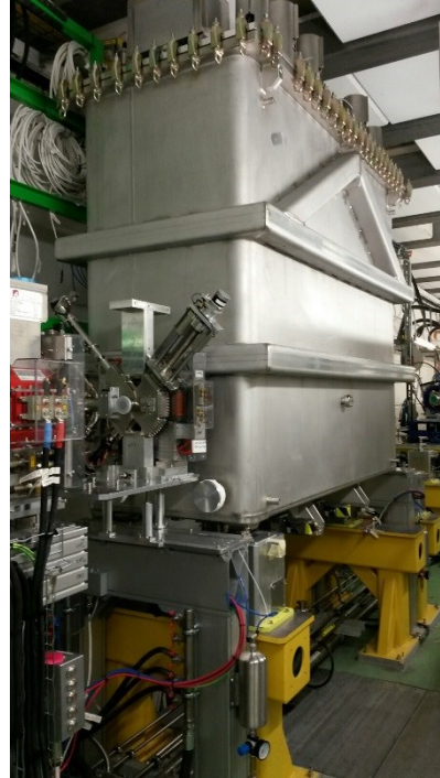
Fig. 10: Cryomodule 2 being connected to its services in the HIE-ISOLDE shielding tunnel
